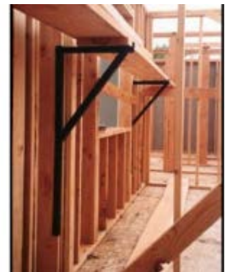
Example 3. Interior scaffolding.
