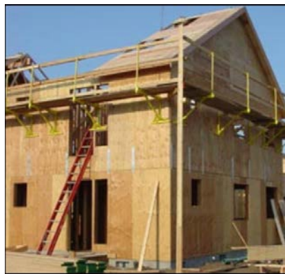
Example 2. Exterior scaffolding on structure.
