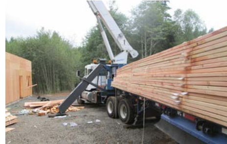
Figure 3. Truck-mounted crane with trusses on the trailer
